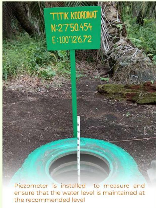
Piezometer is installed to measure and ensure that the water level is maintained at the recommended level
