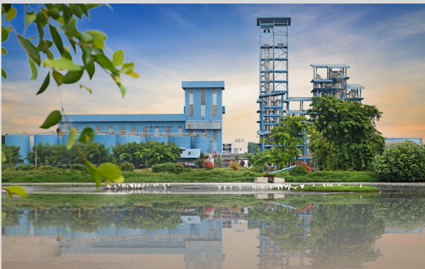
A wastewater treatment plant in one of our units
