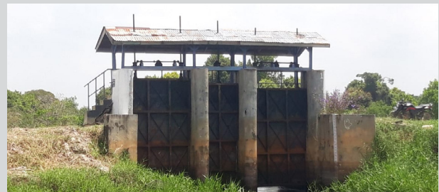
We install water gates to control the water level in our peat area
